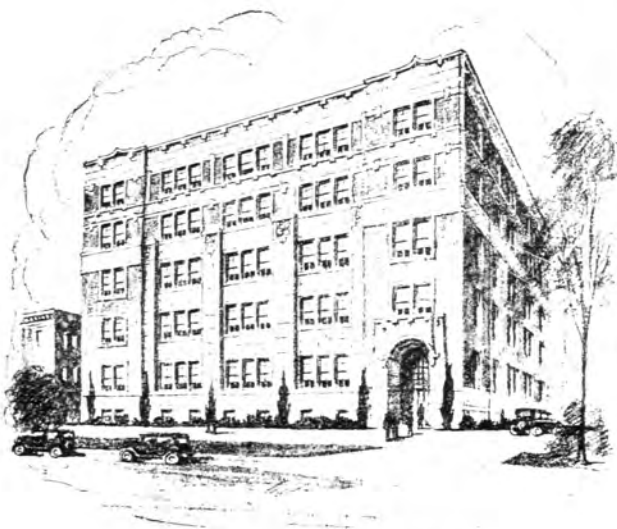
MUTUAL BUILDING LANSING, MICHIGAN
