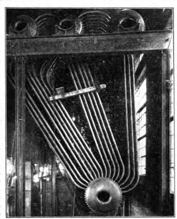
813 H. P. Wickes Four Drum Curved Tube Boiler in process of erection at Michigan State College
